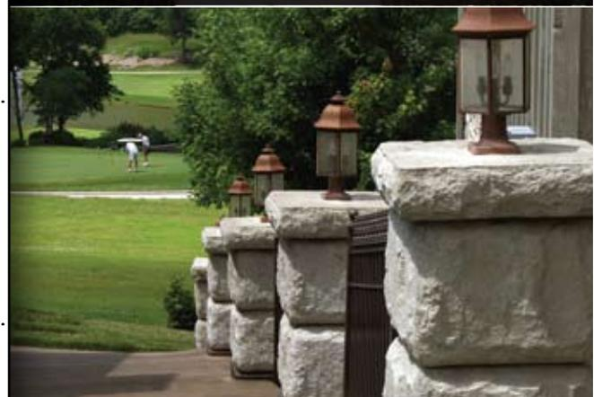
Redi-Rock columns give you the flexibility you need to design the project of your dreams—including the ability to incorporate lighting. The 8 in. core in each block makes it simple.
